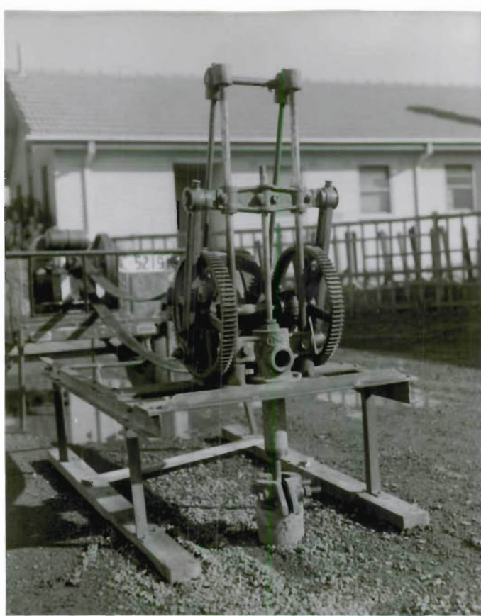
Plate V: Type A.26, Double-gearred Pumphead for Jack pump
