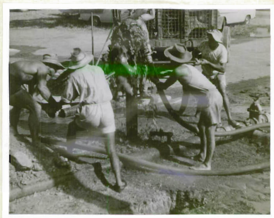
1. Cairns sewerage, trench digger operating between lines of spear-point pumps
