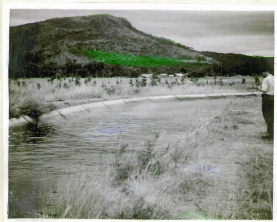
2. Mareeba-Dimbulah Irrigation Scheme, shewing concrete lined trapezoidal channels.
