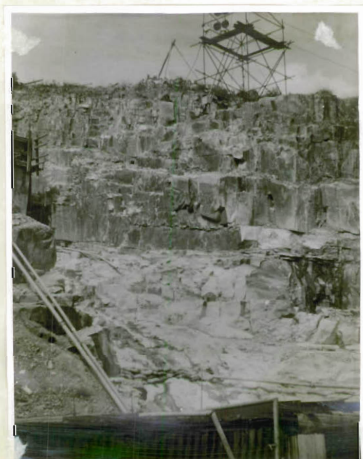
2. Moogerah Dam - Jointing on right abutment.
