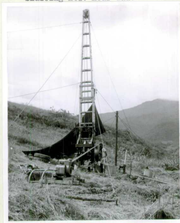
Figure 2A: Close-up Overall McCray percussion drill showing native crew.
