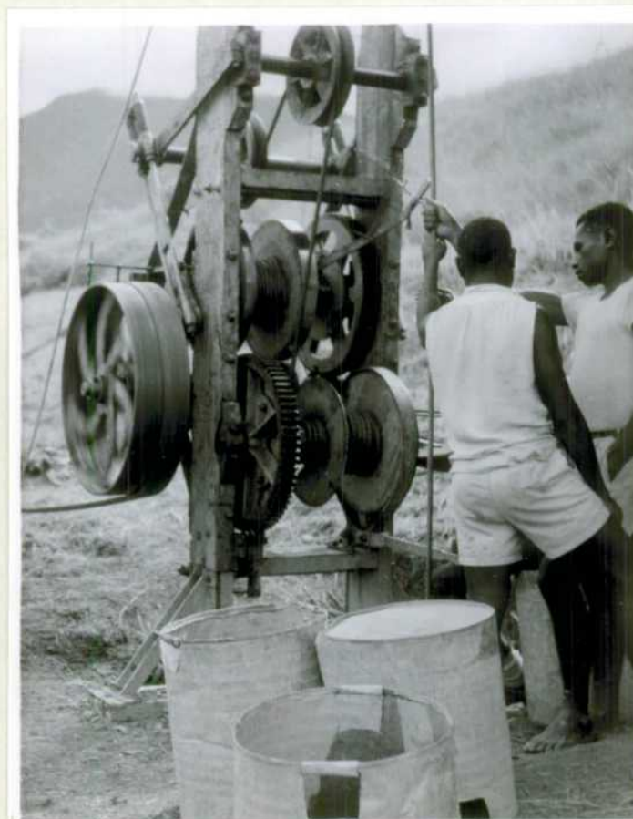
Figure 2A: Close-up Overall McCray percussion drill showing native crew.
