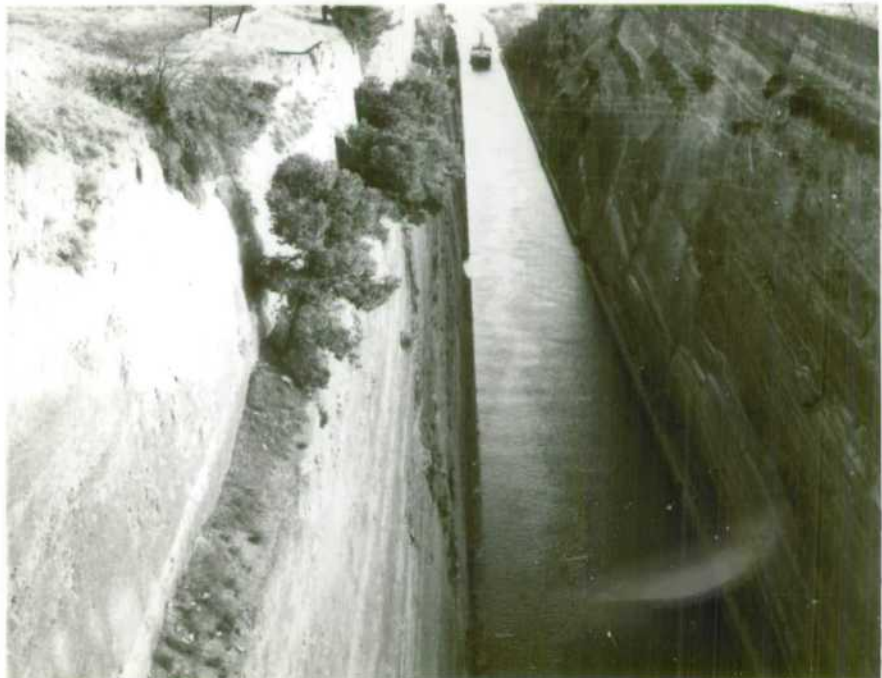
Figure 5. The Corinth Canal cut in faulted Quaternary sediments. The canal links the Aegean and Ionian Seas; it is 4 miles long and depth to water surface in foreground is about 400 feet.
