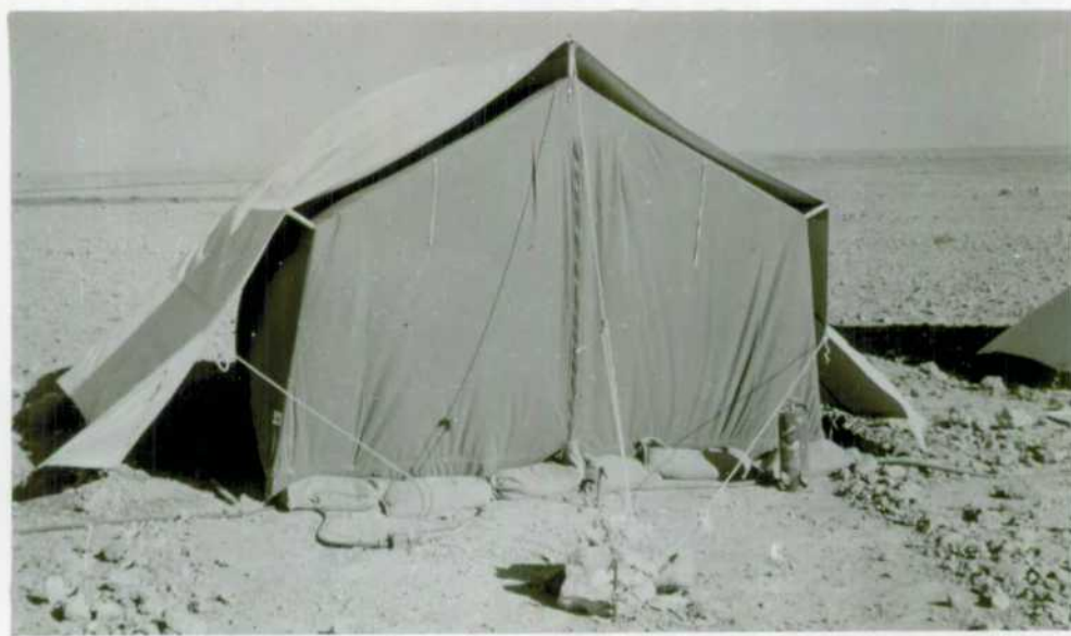
Figure 9 CGG personnel tent and fly are supported by a collapsible frame of galvanised tubing. Both ends of the tent have canvas walls zippered in the centre as above. These walls can be rolled up to reveal inner mosquito netting walls which also have a zippered opening in the centre. The rubberised-canvas floor mat is firmly fastened to the tent wall all round, thus giving good protection from blowing sand and dust.
