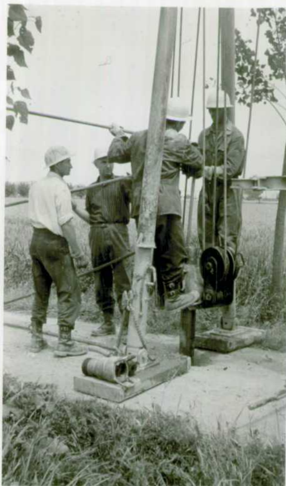
Figure 16 'Spudder' percussion drilling. Charge being loaded inside drill pipe. Tackle is ready for withdrawing pipe after shot.
