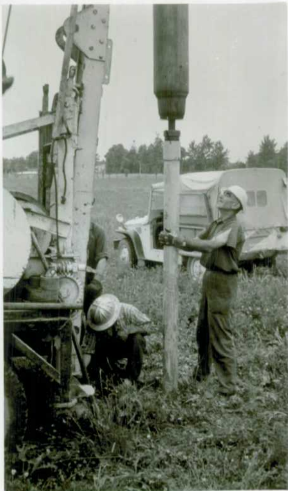
Figure 15 'Spudder' percussion drilling. Note guiding rod and striking plate for percussion weight.
