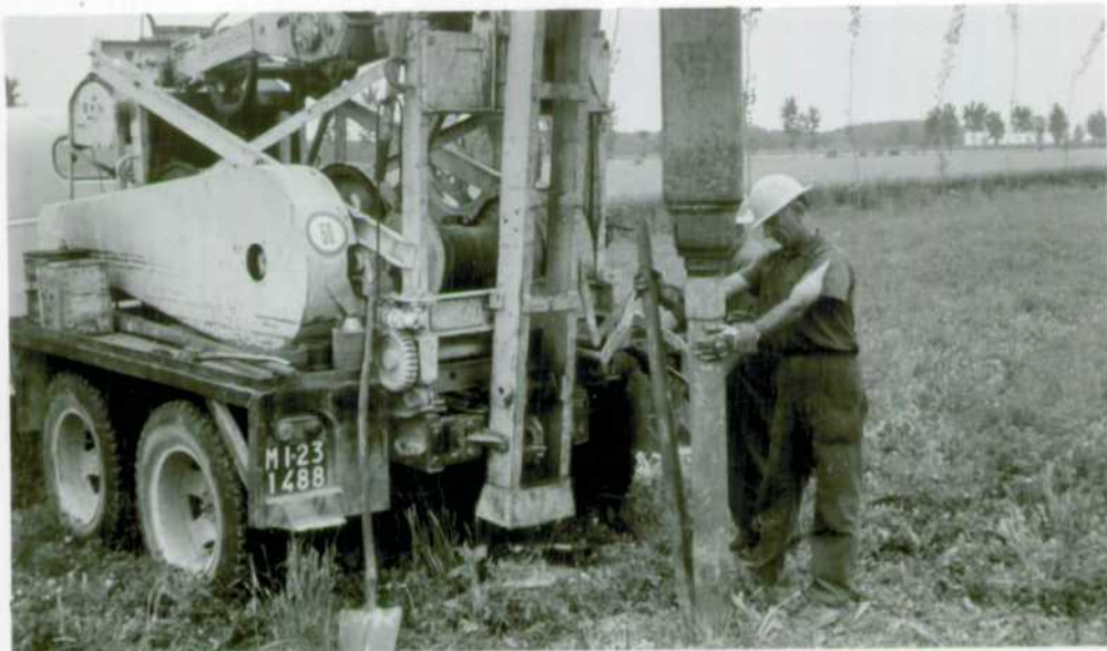
Figure 13 'Spudder' percussion drilling, Po Valley, Italy. Percussion weight hitting drill pipe.
