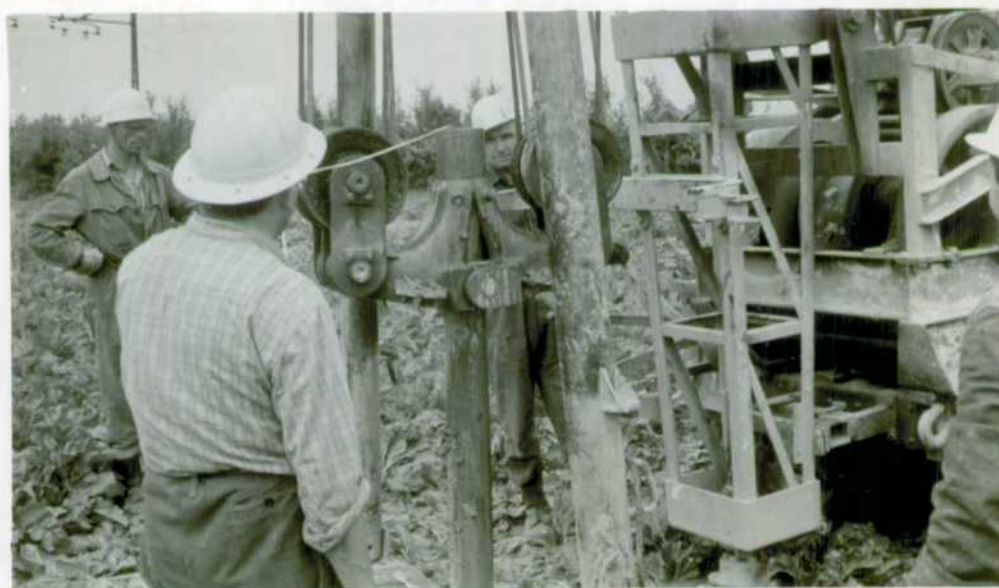
Figure 14 'Spudder' percussion drilling. Photograph shows tackle for withdrawing drill pipe supported by a large 'A' frame. Firing line is seen protruding from drill pipe
