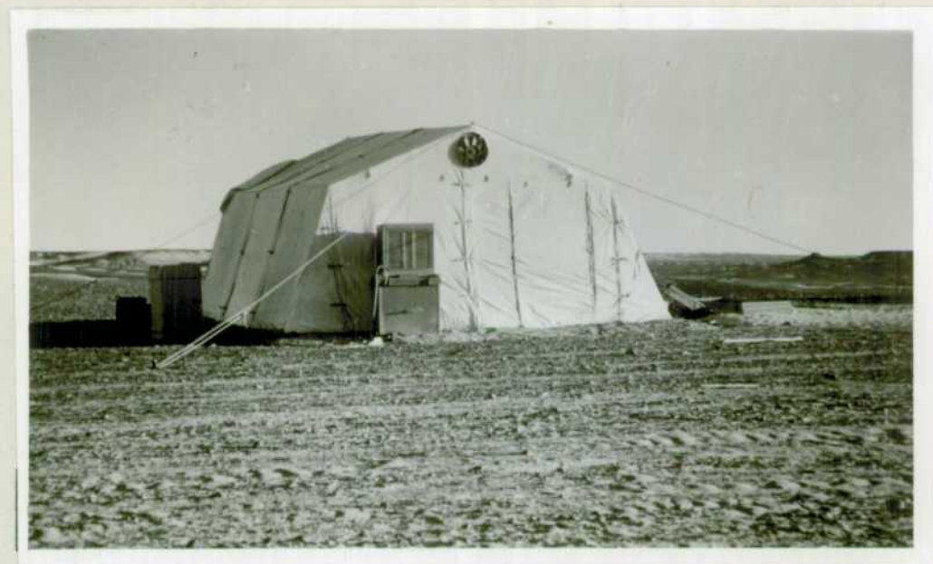
Figure 11 Evaporation-type air cooler and exhaust fan fitted to a large tent used as daytime sleeping quarters in the Central Sahara.
