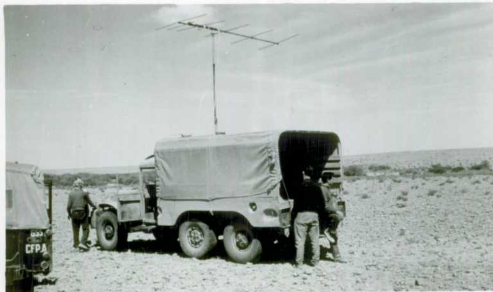
Figure 6 Shooting truck on CGG refraction party, showing VHF radio aerial. This type of radio communication has proved very effective in the Sahara.
