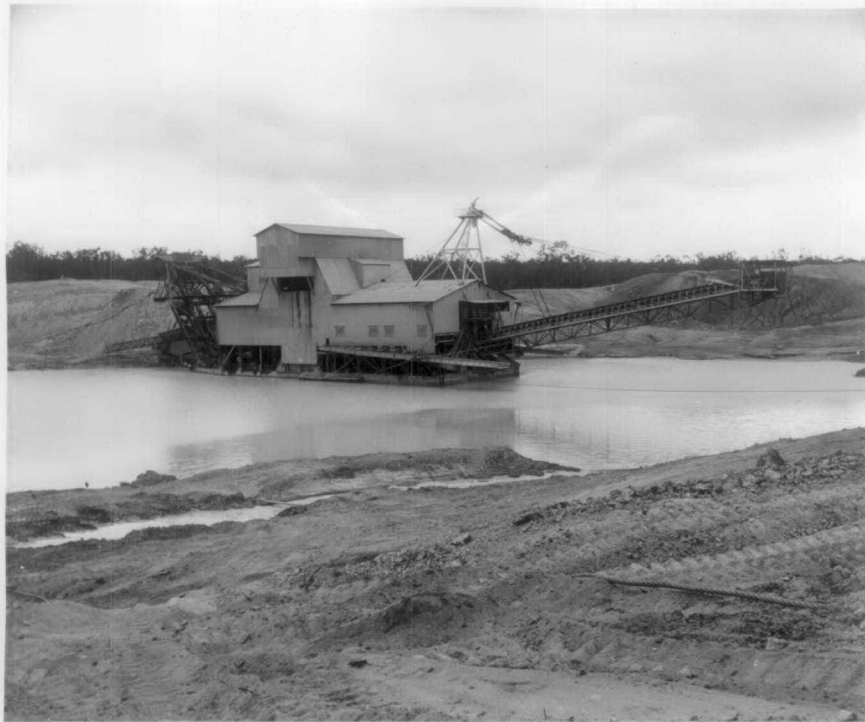
Fig. 20. Tableland Tin dredge, Smith's Creek. Note that the overburden here has been removed by dry stripping.
