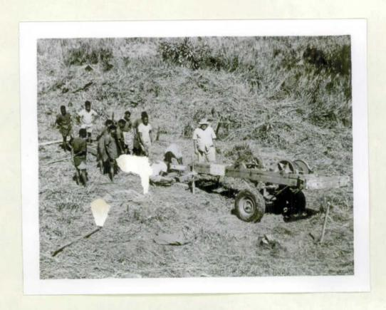
Fig. 1. Assembling Overall-MacCray Percussion Drill.
