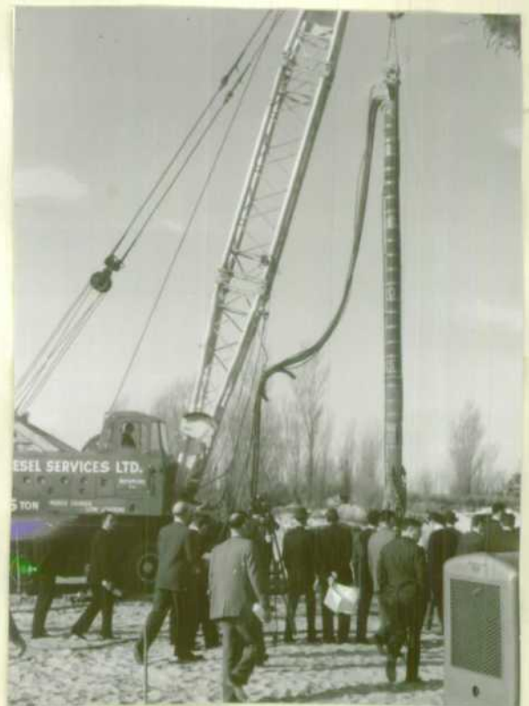
(iv) Vibroflotation equipment
