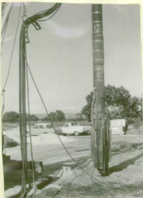
(i) Vibroflotation probe ready to descend.
