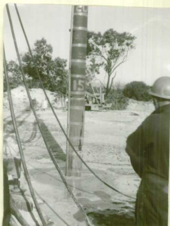
(ii) Vibroflotation probe (10 feet) descending - water is from jets near head of probe.
