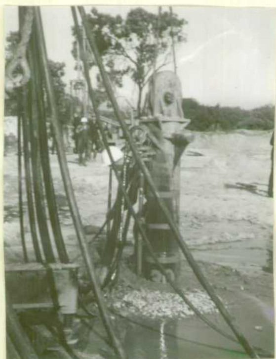
(iii) Vibroflotation probe down 30 feet - rubble surrounding probe is backfill material that is pushed into hole as probe is withdrawn.
