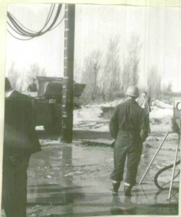
(iv) Vibroflotation probe being withdrawn - front-end loader carries backfill to the probe.
