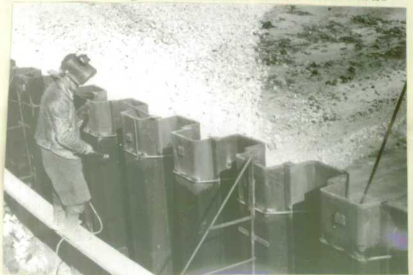
(ii) Sheet steel piling - Bulk handling wharf Port Adelaide.
