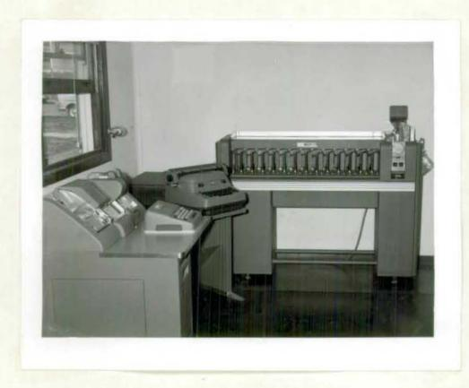
Figure 44: The 870 Document -Writing System on the left of the photograph; the D82 sorter - selector in the background.
