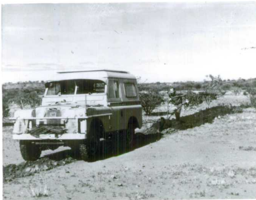
Fig. 3 : Trenching using a modified plough.
