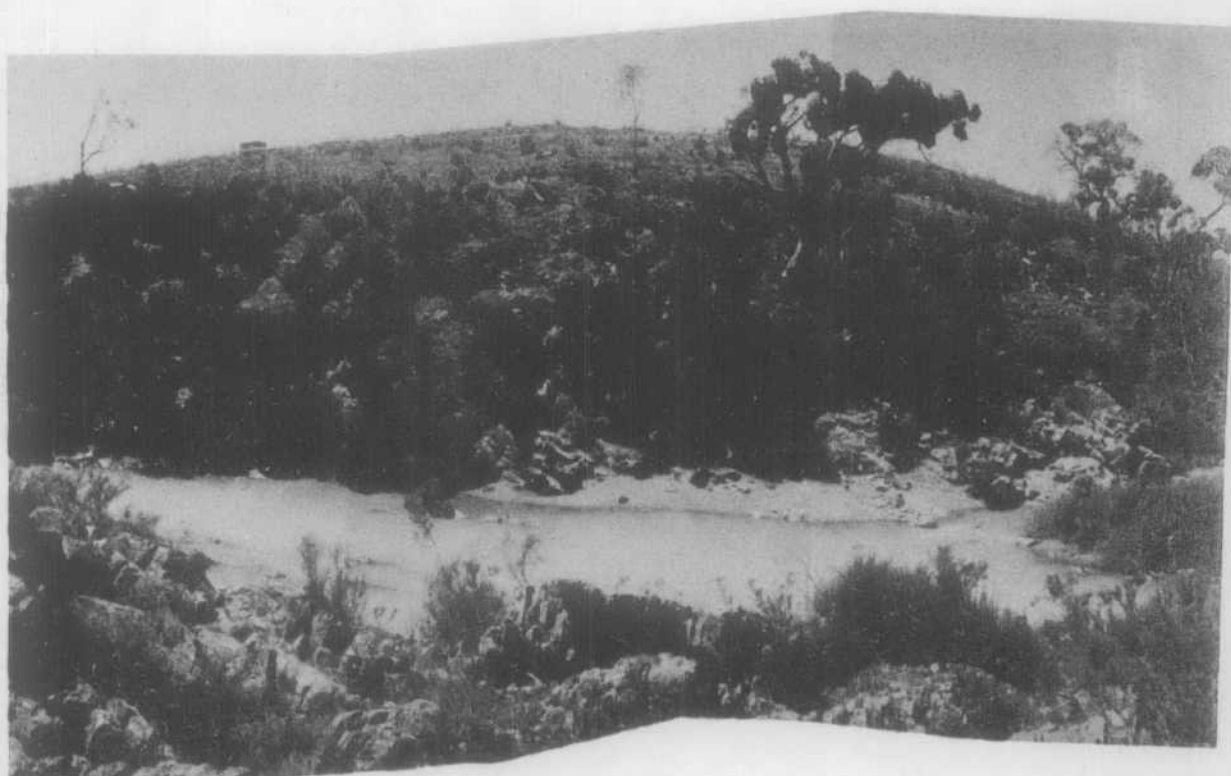
Fig. 2: View of north bank and part of massive sandstone near river on south bank. Plunge of folds in foreground is about 28^{\circ} away from camera. Proposed dam axis passes along a line running from apparent top of hill to bottom left hand corner of photo.
