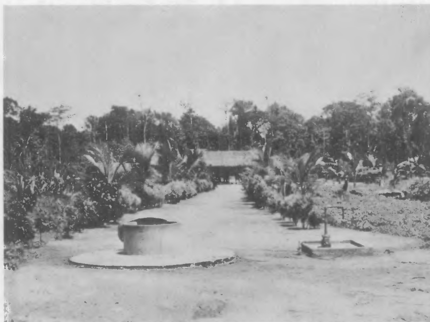
Plate 2B. Standard Sanitary Well at IDOLI village, West Sepik District. The cement cover for the well has been removed for inspection.
