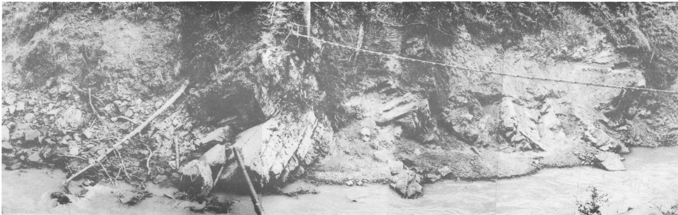
Figure 12: Left abutment of weir site No. 2
