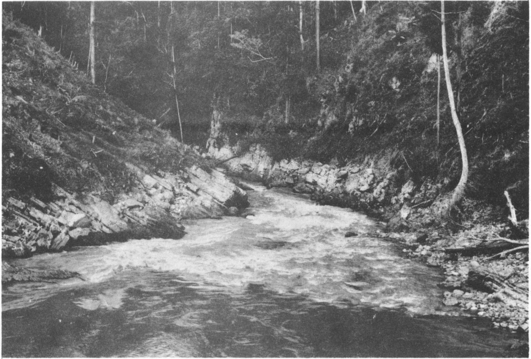
Figure 8a: Weir site No.1, Ramu River, looking downstream. Slope of left abutment is closely controlled by dip of bedding in metasediments.
