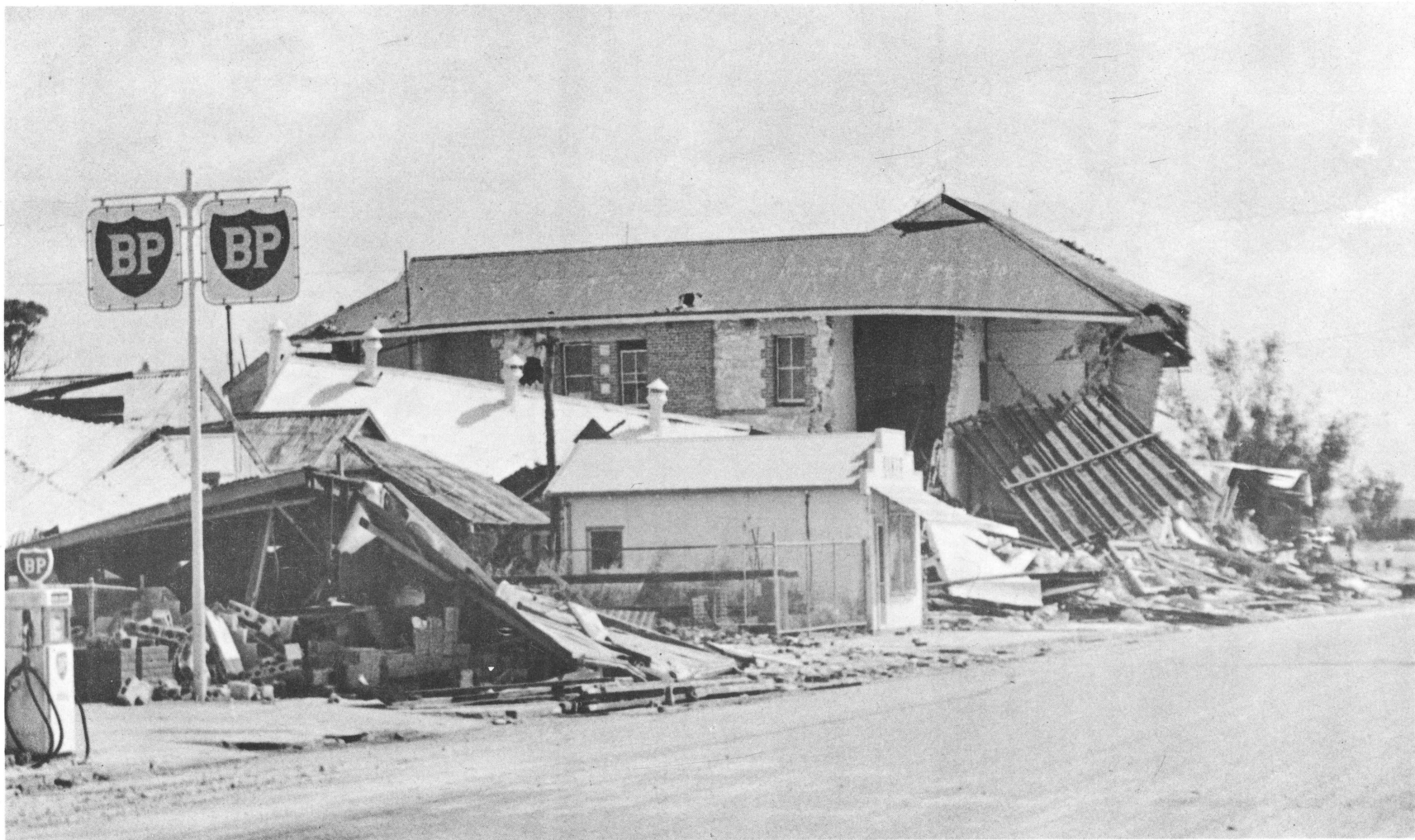
DAMAGE - MECKERING: Fibro-cement baker's shop relatively undamaged
