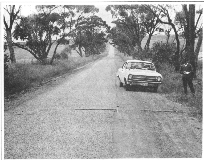
FRACTURE ZONE: (a) Minor transcurrent fault 1 mile east of major fracture; 7 miles south of railway, looking south. (note en-echelon faulting)
