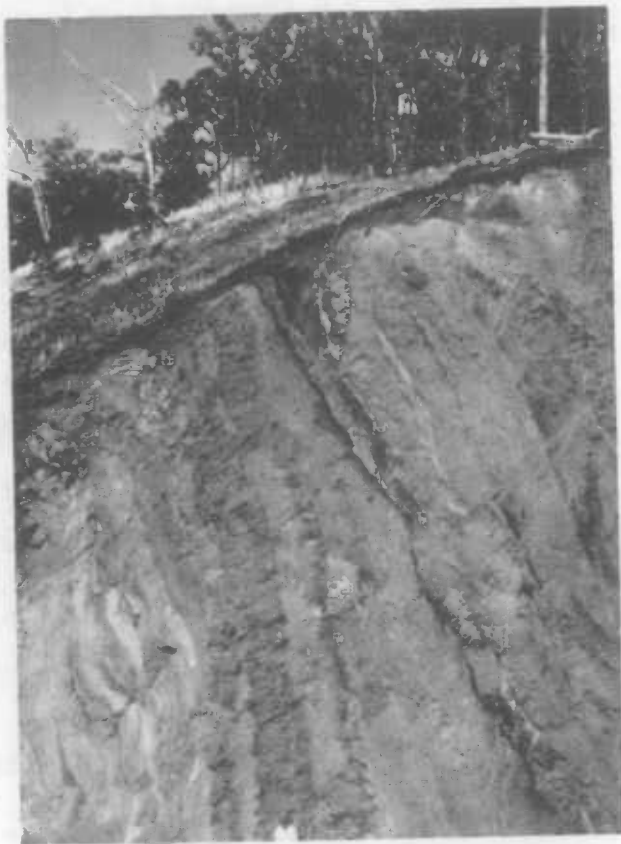
Road cutting on the Cunningham Highway through steeply dipping Walloon Coal Measures; note disrupted coal bands and Tertiary basic sills (grid ref. 554520)
