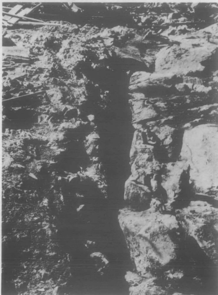
Fig. 12 :- Views of Fault E exposed in the valley floor core zone foundations. The top view shows the fault after sluicing of the bedrock surface; the bottom view shows the extent of excavation for concrete dental treatment. Approximate co-ordinates of the centres of both views are 540 E, 985 N.
