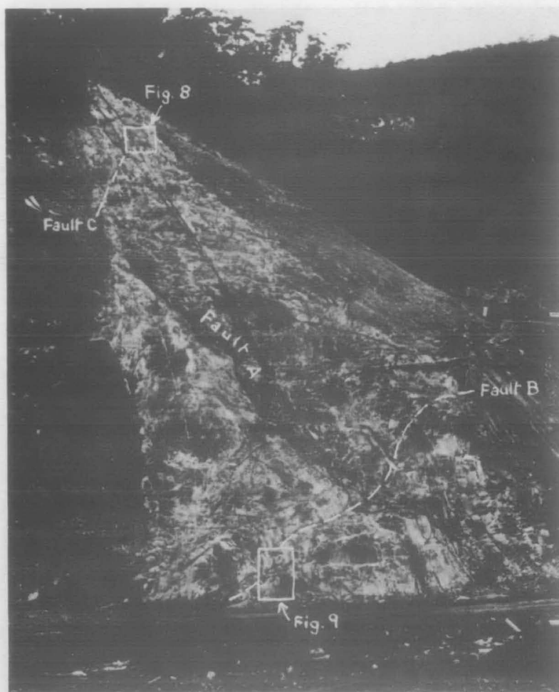
Fig. 7 :- The eastern core zone foundations, after removal of overburden by sluicing, showing the prominent surface trace of Fault A, and the positions of Faults B and C.
