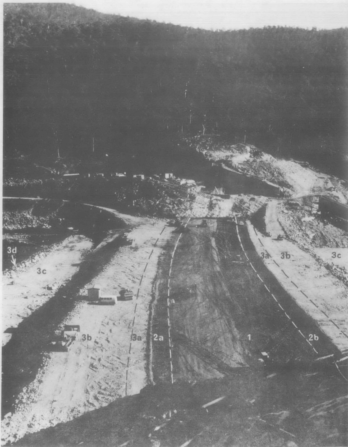
Fig. 3 :- Photograph of the dam during construction showing the zoning of construction materials - see Fig. 2 for descriptions of the various zones. The top of the core zone is at R.L. 3068 feet.
