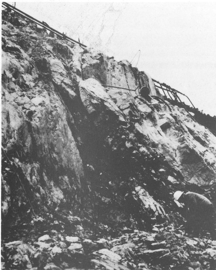
Fig. 9 (a) :- Fault B (dipping 70^{\circ} to the west) as exposed in the eastern core zone foundations after removal of overburden by sluicing. This view is taken from the downstream boundary of the core zone (see Fig. 7).
