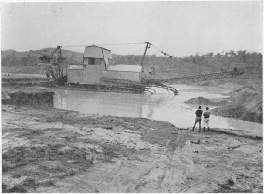
Plate 16, fig. 1. Dredge operated by Tableland Tin Dredging NL in Smiths Creek, west of Mount Garnet.
