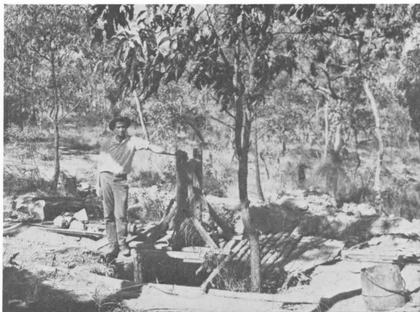
Plate 15, fig. 1. The Rover tin mine, South Coolgarra, a typical example of one of the smaller mines in the Herberton Tinfield. In June 1968, when the photograph was taken, the main shaft was 23 m deep. The mine is in Elizabeth Creek Granite.
