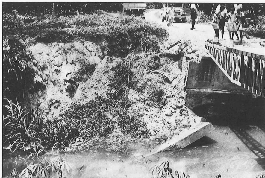
Failure of abutment, Murnase River bridge. Typical of failure at smaller bridges.
