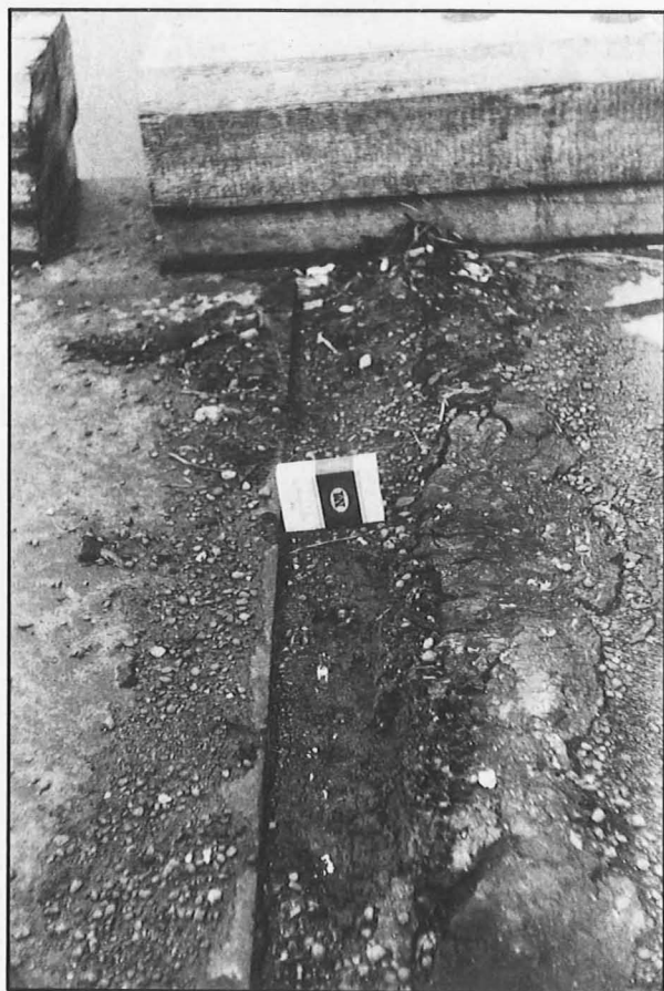
Madang wharf movement. Relative movement between mainland and Madang main wharf (at right) about 8 cm. evidenced by bitumen scraped off wharf by steel plate (left).
