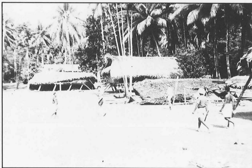
Typical village wrecked by earthquake. About 50 per cent of houses were wrecked where intensity was MM8 or more.
