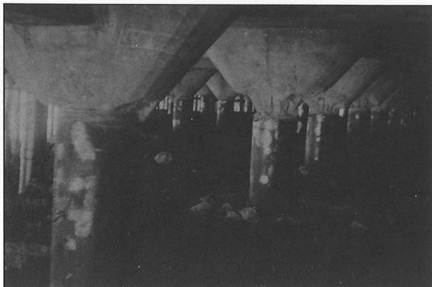
Madang wharf damage. Spalled concrete due to formation of plastic hinging at the top short piers at rear (landward) side of wharf.
