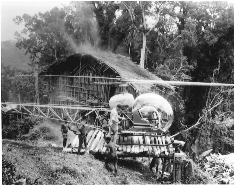
Figure 2: Helicopter pad constructed by a Bureau of Mineral Resources traverse party (one geologist and five carriers) at the end of a week-long traverse in the headwaters of the Salumei River, South Sepik region. It was not always possible to find clearings at the end of a traverse, and often a full day's work was required to clear a pad in virgin forest.
