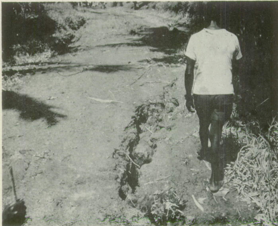
Figure 10. Cracking typical of built up road edges, Buin-Koniguru road.
