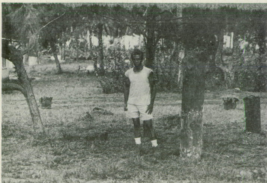
Figure 15. Old wharf piles at Torokina extruded by the effects of liquefaction caused by aftershocks. The tops of the piles were formerly below ground level, as indicated by the grass and plants growing on them.
