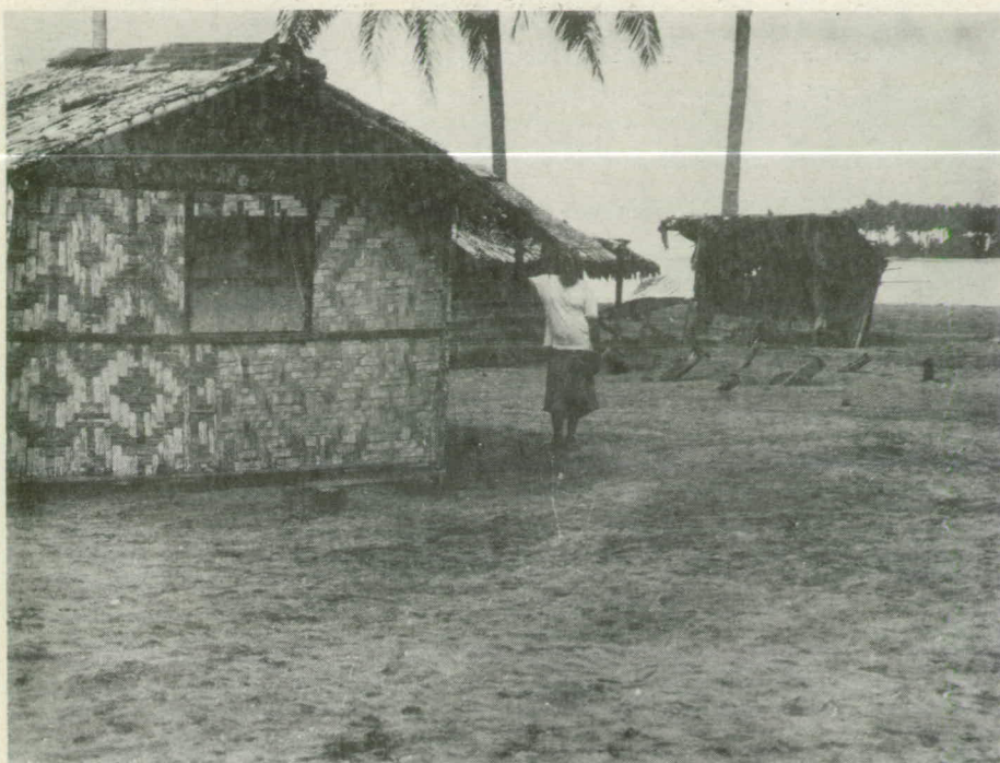
Figure 12. Village house removed from stumps (in centre of picture) by tsunami, Torokina.
