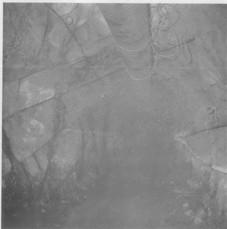
Fig 16 : Pine Ridge Tunnel, stn 62 + 70. Joints (? bedding) in blue grey dacite. (RCN 3-4).
