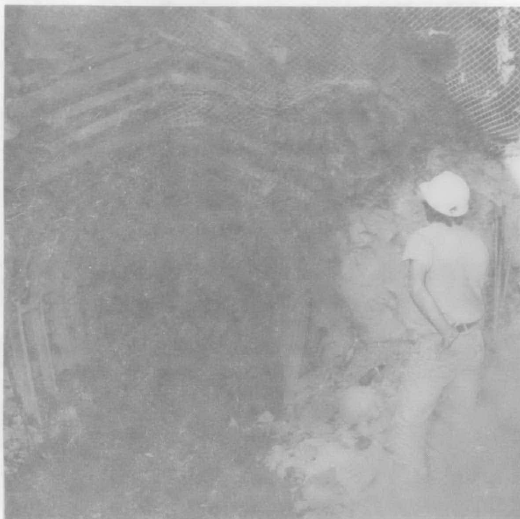
Fig 13 : Ryan Tunnel inlet portal - large overbreak with support and logging; mesh and rock bolts around the portal.
