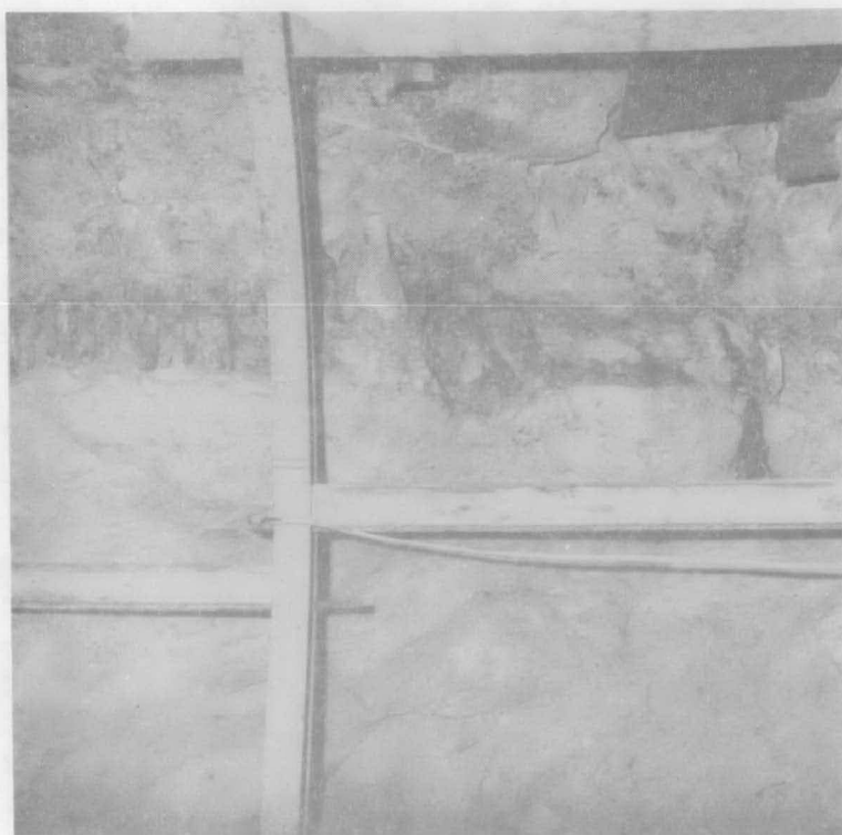
Fig 14 : Ryan Tunnel, stn 47 + 20 west wall, showing dark green olivine dolerite sill in rhyolite agglomerate. (RCN 4-5).
