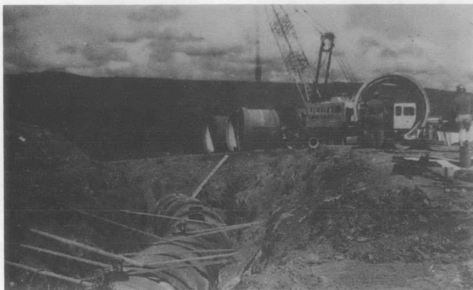
Fig 17 : Pipe-laying in Mount Painter Porphyry near Coppins Crossing Road. (M2256/4)
