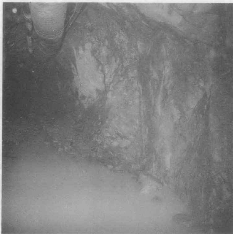
Fig 15 : Ryan Tunnel, stn 46 + 20. Overbreak in wall as a result of planar slickensided joints in grey dacitic agglomerate. (RCN 3-4).
