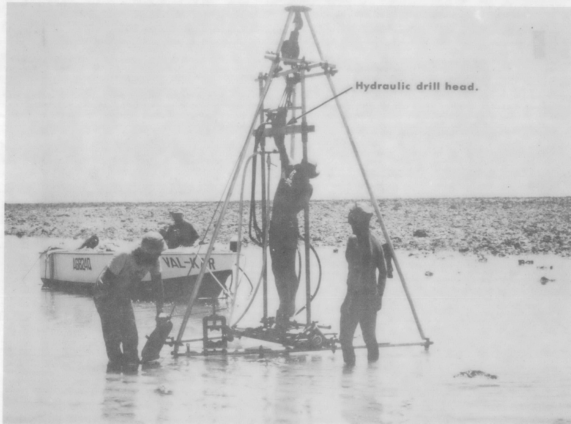
FIG 4-12-2 HYDRAULIC ROTARY CORING DRILL
