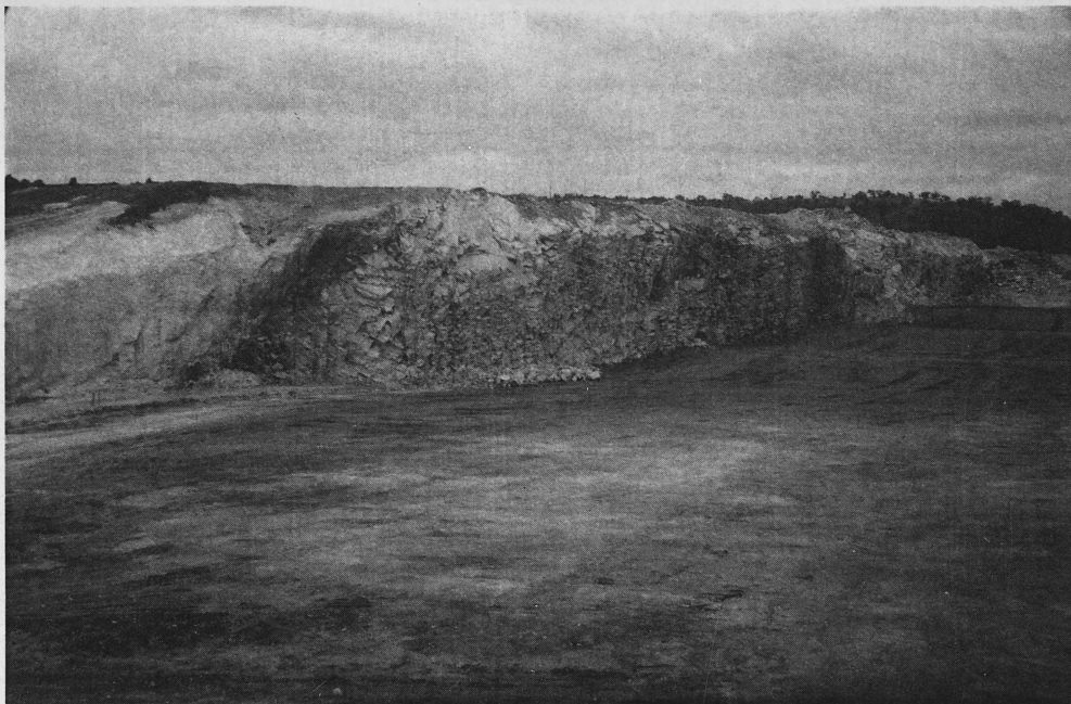
Fig. 7. View of completed rock face on eastern side of central excavation at northern end. Dark patch on face at left centre is ferruginous fault zone (Fault A) separating white, leached siltstone of Canberra Formation at extreme left from Black Mountain Sandstone.
