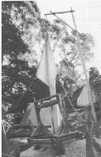
As the deep lead mines got deeper, the miners often encountered bad air. The Windsail was the method they used to get clean air into the mine. The idea came from sailing ships where scoops were set up to get clean air into the bottom of the ship.
