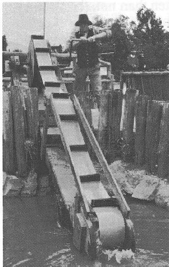
Miners needed water in the processes used to extract gold and sometimes they had to move water uphill. Using buckets could be very tiring. This slide shows a California Pump. Small boards are connected to a leather belt around two pulleys and the bottom end is placed in the water. The pump required a man to turn the handle to pull water up a wooden tunnel.
