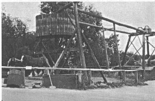
After 1854, mining rules were changed to allow for bigger claims to be worked by groups. As a result, diggers joined together to make mining easier and so they that could buy or make equipment using more advanced technology. On the Whim, one bucket lifts up the shaft while the other bucket is let down. A wire is wound from one bucket, over a pulley, around a drum, over another pulley and down to the other bucket. Because the miners used huge containers, the whim could bail 300 gallons
