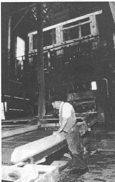
This machine operates at Sovereign Hill to crush quartz to release the gold inside. A steam engine turns the cams which lift the stampers. A labourer shovels quartz into the stamper box at the bottom where the heavy stampers fall to crush the rock. Water then carries the crushed rock, as sand, over mercury plates where most of the gold forms an amalgam with the mercury. The sludge left over then flows over a corduroy blanket where any remaining heavy gold is caught in the corduroy.
