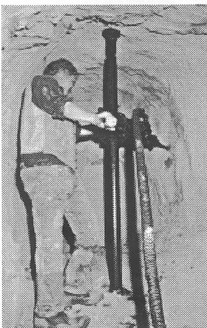
This drill was driven by compressed air made by a steam engine. The air was fed through pipes to the drill in the mine. The drill was used to bore holes in which explosives were laid to break away the rock face. This machine was also known as "The Widow Maker" because the dust it created caused a disease called Silicosis or "Miners' Lung" which eventually killed many miners. Many miners also went deaf because of the noise of this machine.
