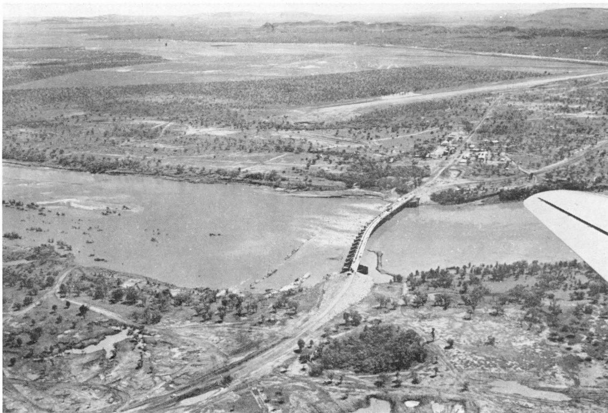
Plate 1. Aerial view, looking northeast, of the Ord River diversion dam, taken in wet season during construction. The dam rests on a bar of Precambrian quartzite, Bandicoot Bar. Kununurra is on the right of the field of view, in front of Kellys Knob and the sandstone scarp which is visible up to Abney Hill. Behind and to the left of Abney Hill is the Pincombe Range. The dome on the right-hand skyline is Mount Cecil
