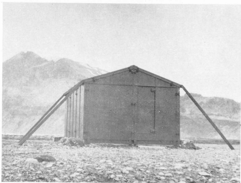
Fig. 2. Variometer hut, looking north-west
