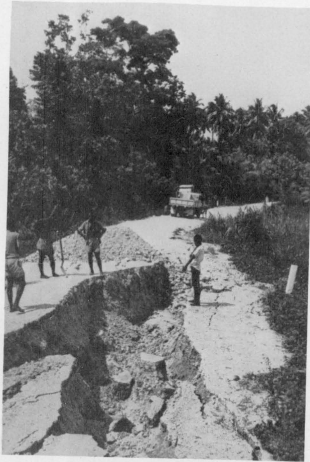
(a) Slumping and settling of the Surumarang River bridge approach — typical outcome of built-up sections of roads near bridges where MM7 or greater intensity occurred. The six-metre-high built-up approaches to the Gogol River bridge settled two metres.
