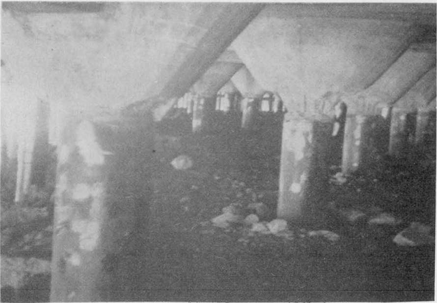
(b) Madang wharf damage. Concrete spalled by plastic hingeing at the top of the short piers at the landward side of the wharf.
