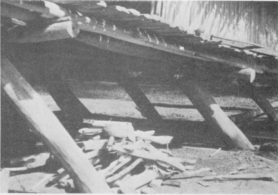
(a) Floor and stilt structure of village house. Note that the stilts are not tied to the flooring, nor are they braced. The stilts sag north-northeast, transverse to the direction of the epicentre.
