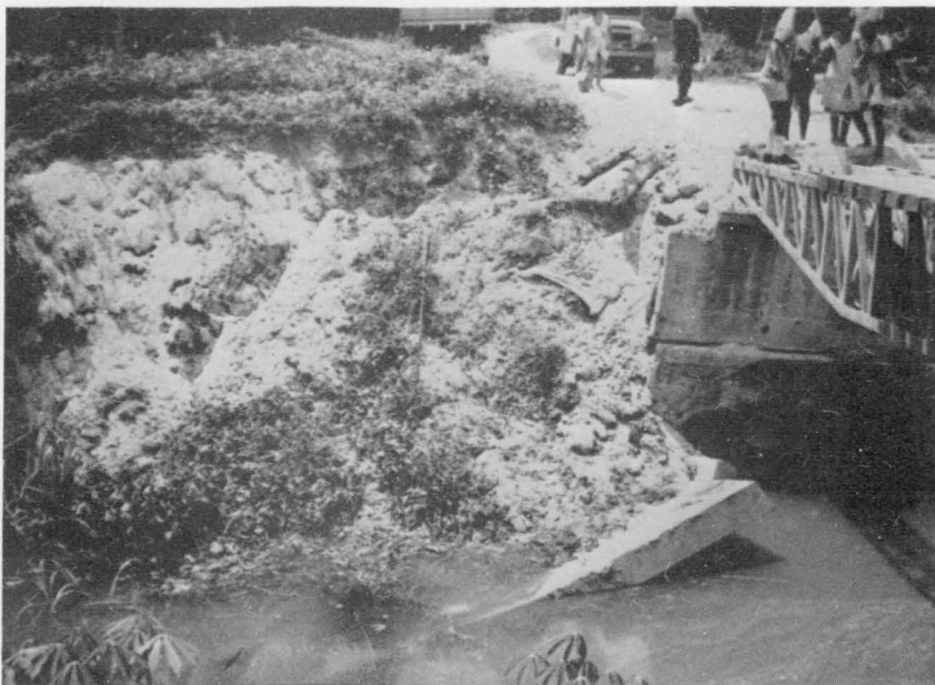
(a) Failure of abutment, Murnass River bridge — typical failure of smaller bridges.
