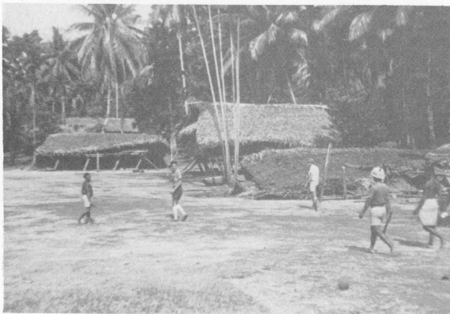
(a) Typical village wrecked by earthquake. About 50 percent of houses were wrecked where intensity was MM8 or more.
