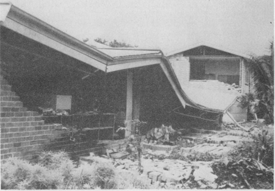
(a) Lightfoot Arcade, Madang. Note that the wall has fallen outwards, and the roof is held up by shelving in the centre of the photograph.
