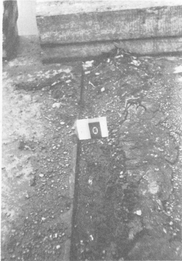
(a) Madang wharf movement. Relative movement of about 8 cm between the mainland and Madang main wharf (at right) is evidenced by bitumen scraped off the wharf by the steel plate joined to the mainland.
