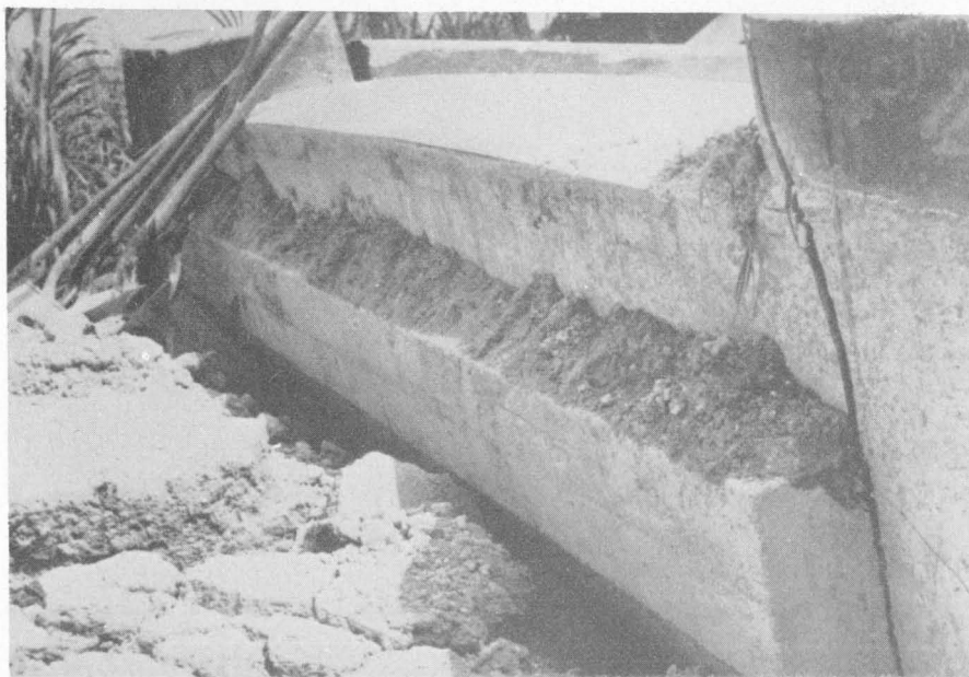
(b) Surumarang River bridge thrust against northern abutment. Note the settling of the built-up approach (left) previously level with the top of the abutment. The bridge runs transversely to the direction of the epicentre.
