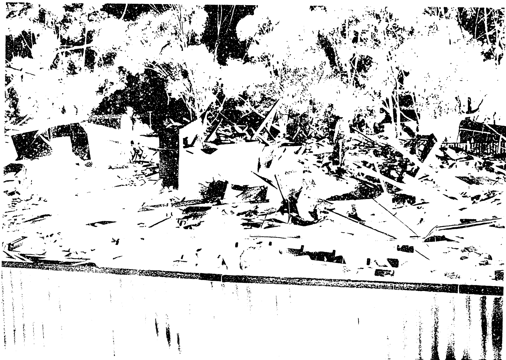
13 Damage to cement brick house, adjacent to northern fracture zone.
