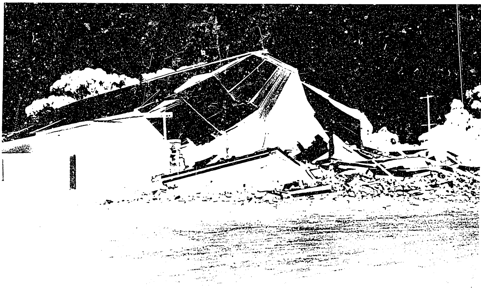
16 Damage to public hall. Collapse of brick front.
