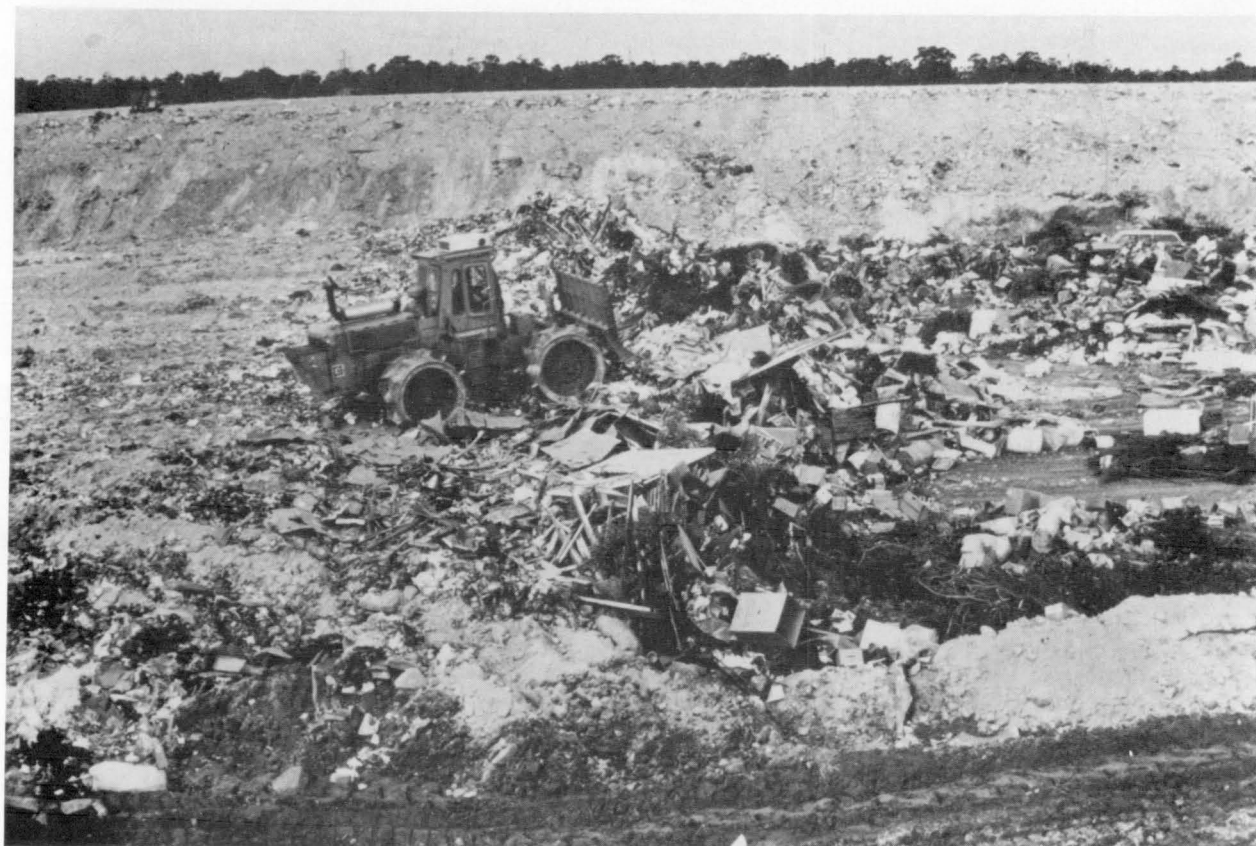
Fig. 7. Heavy compactor in use at the Lucas Heights Regional Waste Disposal Depot, Sydney.
