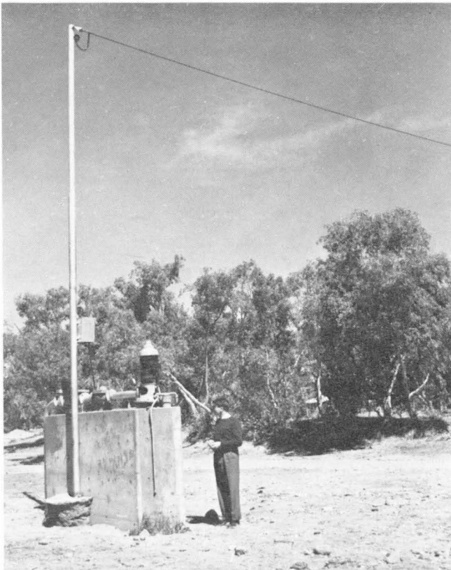
Fig. 2. Bore 62/9, in bed of Todd River, showing concrete pier installation to raise pumping equipment above level of river flows (Photo: J. Zawartko)
