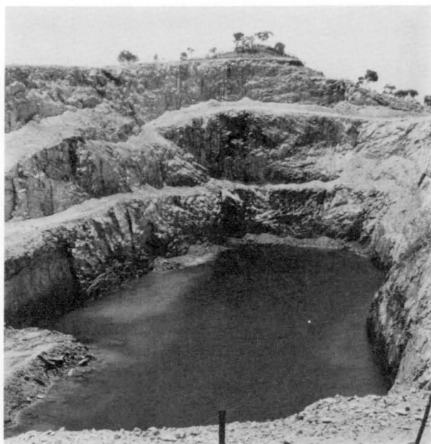
Fig. 78. Open cut of the Young Australia copper mine, 5 km southwest of Kuridala (at GR VB383403). The lode was situated in a steeply dipping, north-trending, kaolinised fault zone, and contained malachite, chalcocite, cuprite, tenorite, and hematite (Donchak & others, 1983). Photograph taken in 1980. (M2491/3A)
