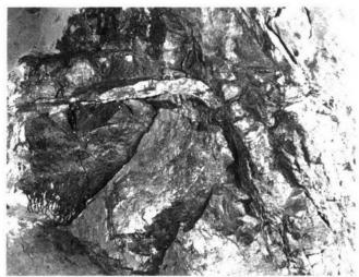
Figure 18.3. Faulted quartz vein (reef) in the Bushmans Hill gold mine, Parkes. The vein has been dragged downwards into the fault on the right hand side, indicating normal displacement. (Photo taken in July 1897, DMR collection, Forbes 0012).
