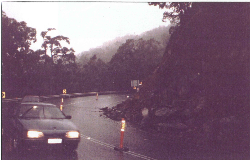
Plate 11. Rain on 26 February 1999 triggered this 500 cubic metre rock topple/fall near the Smithfield end of the Kuranda Range Road. The landslide was still active the next morning, when this photo was taken.
