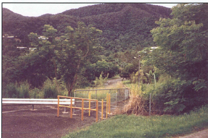
Plate 8. During Tropical Cyclone 'Joy' in December 1990 a landslide to the left of the steel fence in the centre foreground severed the traffic connection between Granadilla Drive in the foreground and Comet Street, Bayview Heights, near the centre of the photo. The two roads are now connected by only a footpath.
