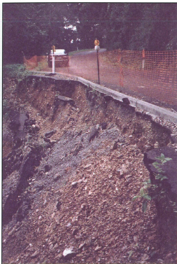
Plate 10. Fill failure on Lake Morris Road, triggered by the heavy rain in March 1999.
