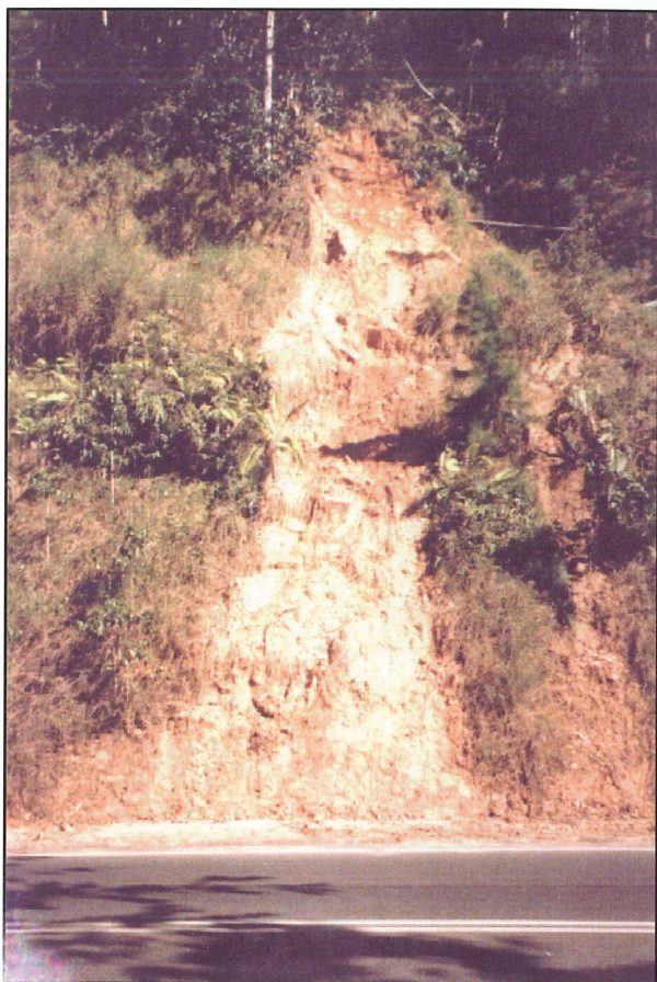
Plate 9. One of 46 batter failures on Kuranda Range Road, triggered by rain brought by Tropical Cyclone 'Justin' in March 1997.
