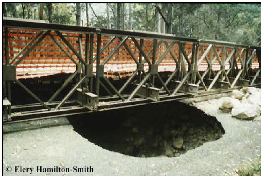
Figure 1 Road collapse due to inappropriate location of road. (Photograph courtesy of Elery Hamilton-Smith)
