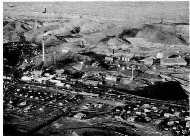
Figure 12. A view of the Mount Isa Ag-Pb-Zn and Cu mines, looking west. The contact between the Judenan Beds and the Mount Isa Group coincides with the Mount Isa thrust fault.
