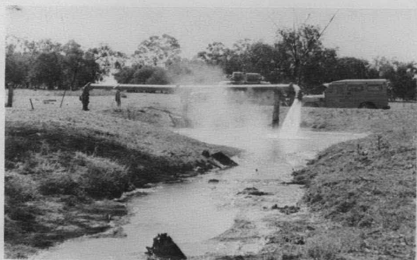
Figure 14. Flowing artesian waterwell in the Great Artesian Basin (WRC-NSW Reg. No. 4263—Four Posts-2; depth 1174 m, flow 35 l/sec, wellhead temperature 57°C; aquifer Pilliga Sandstone).
