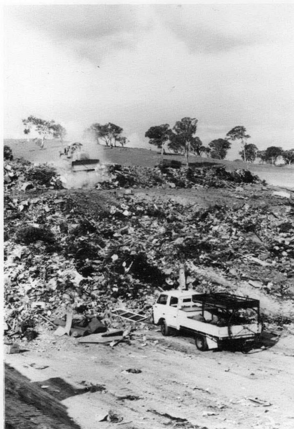
Figure 1. Compaction of solid waste at the Mugga South sanitary landfill site, ACT.
