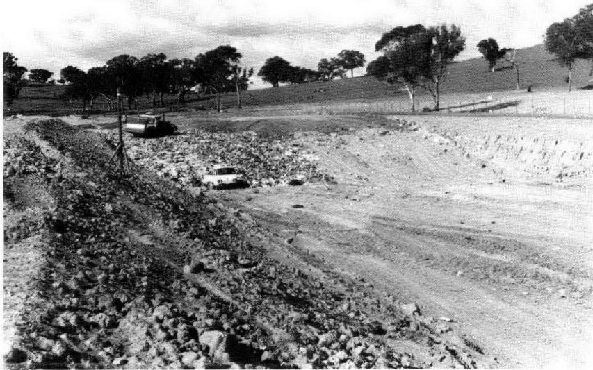
Figure 9. Mugga South sanitary landfill site, ACT, developed on Cainozoic colluvial outwash fan deposits.
