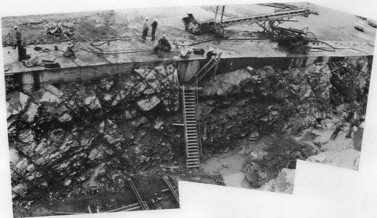
Figure 12. Corin Dam spillway crest foundations, showing overbreak along well-developed 30^\circ joint set. The arrows in the top photograph identify some of the prominent joint faces.
