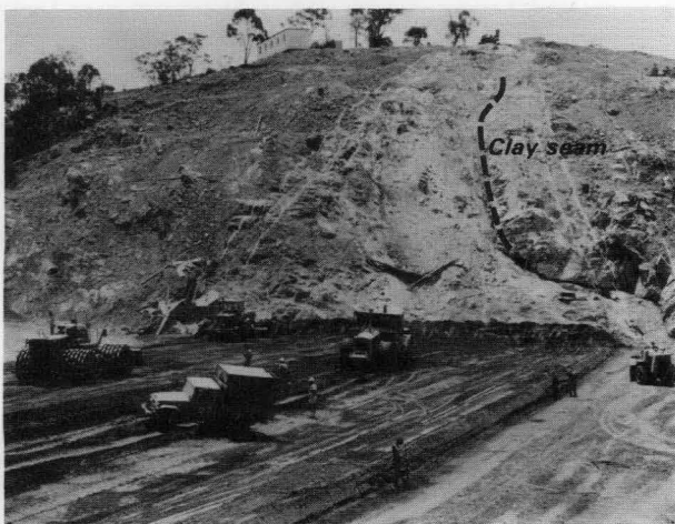
Figure 15. Clay seam in right bank of Geogong Dam foundations.
