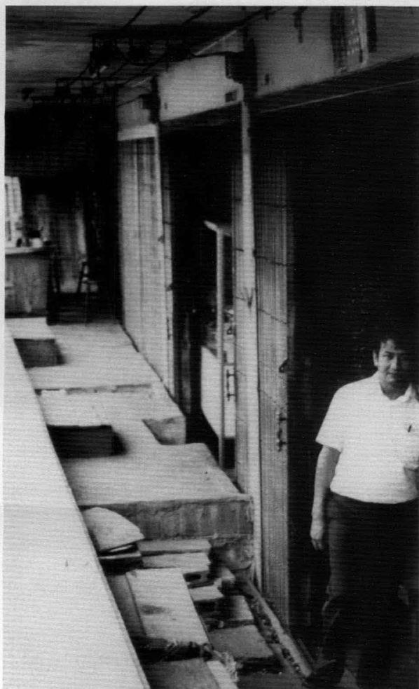
Figure 15. Dramatic evidence of building subsidence in Bangkok as a result of groundwater withdrawal.
