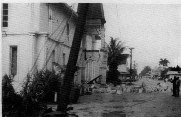
Figure 9. Damage to the Prime Minister's building, Nuku'alofa, resulting from the 1977 Tongan earthquake.
