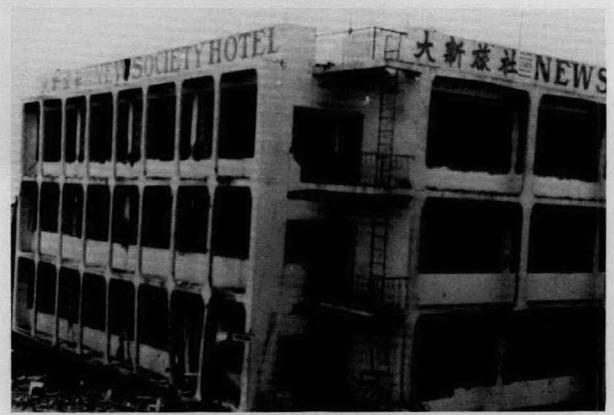
Figure 3. Damage to this Cotabato City hotel was caused by the 17 August 1976 western Mindanao earthquake in the Philippines.
