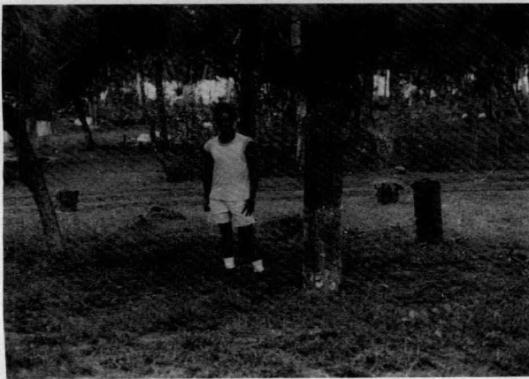
Figure 6. Old piles from a Second World War wharf at Torokina were extruded by the effects of liquefaction caused by aftershocks from the 20 July 1975 Bougainville earthquake.
