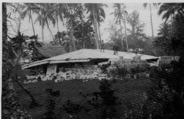
Figure 8. Collapse of a masonry house on 'Eua caused by the Tonga earthquake of June 1977.
