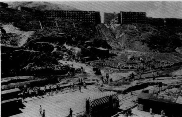
Figure 11. This landslide during the Hong Kong typhoon on 17 June 1972 damaged the retaining wall in front of a new seven-storey apartment building at San Mau Ping and buried a squatter settlement and the inhabitants under 3 m of mud and debris. Photograph by Kin Che Lam. M2689.
