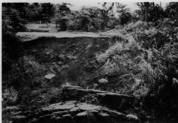
Figure 17. The main coast road between Suva and Nadi on Viti Levu (Fiji) was cut by landslides during Cyclone Wally in April 1980, and was still impassable when this photograph was taken by M.J. Crozier in May. GB3325.
