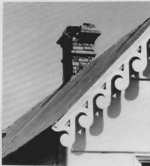
Figure 3. Earthquake-damaged chimney in Lithgow.
