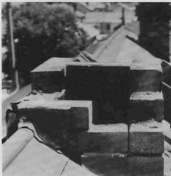
Figure 2. Chimney in Lithgow, collapsed at the roofline because of the earthquake.
