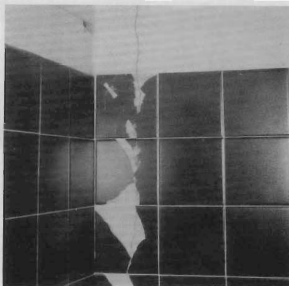
Figure 6. The vertical crack in Figure 5 continues down into the tiles in the lower part of the wall.
