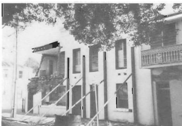
Figure 12. Part of the brick wall in Figure 11 was considered unsafe. It was demolished, and the rest of the wall propped up before repair. Photo: M. Michael-Leiba.
