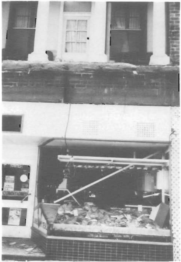
Figure 10. Butcher's shop in Hamilton. The parapet collapsed onto the awning, which fell to the street, showering bricks and rubble over the window display. Photo: M. Maloy.
