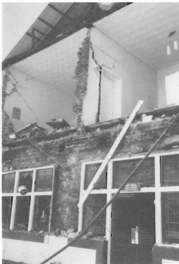
Figure 13. Two storey commercial building, Beaumont St, Hamilton, showing failure of both inner and outer brick walls of top storey and gable. Photo: M. Maloy.
