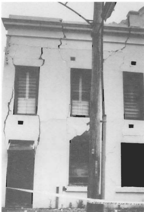
Figure 11. Typical damage in masonry walls, where cracks have formed at stress concentrations at the corners of windows and doors. Photo: M. Maloy.
