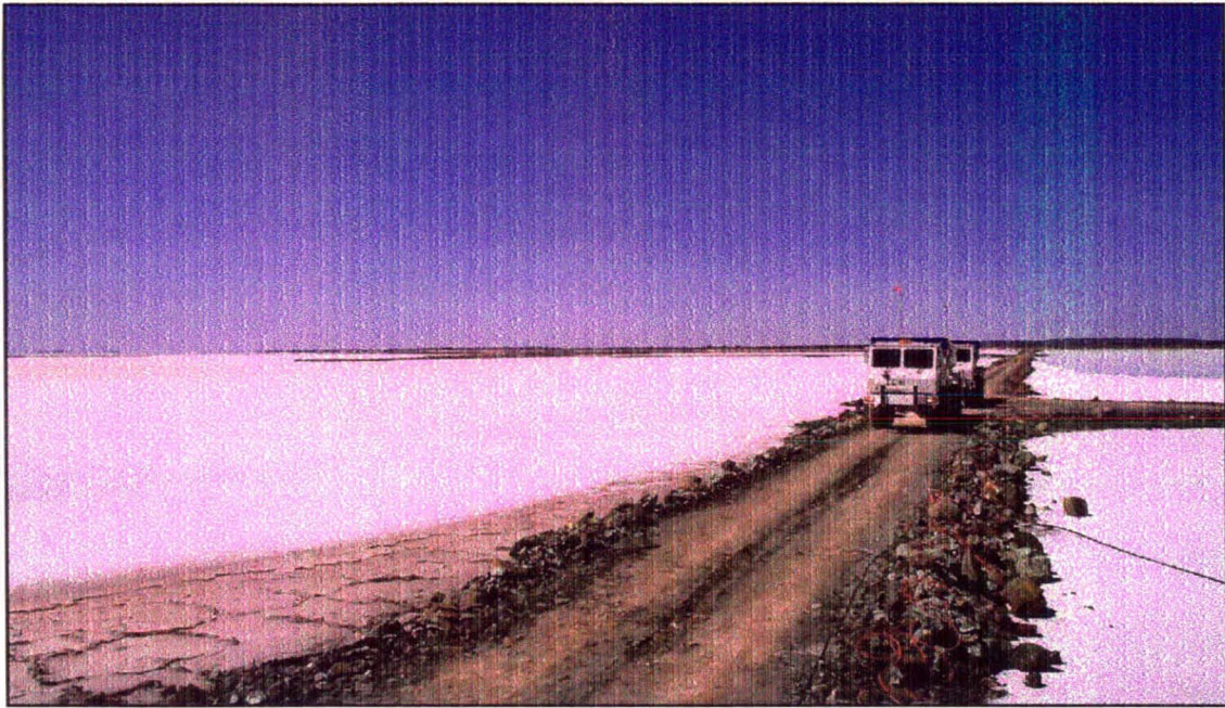
Vibes operating up causeway towards haul road
