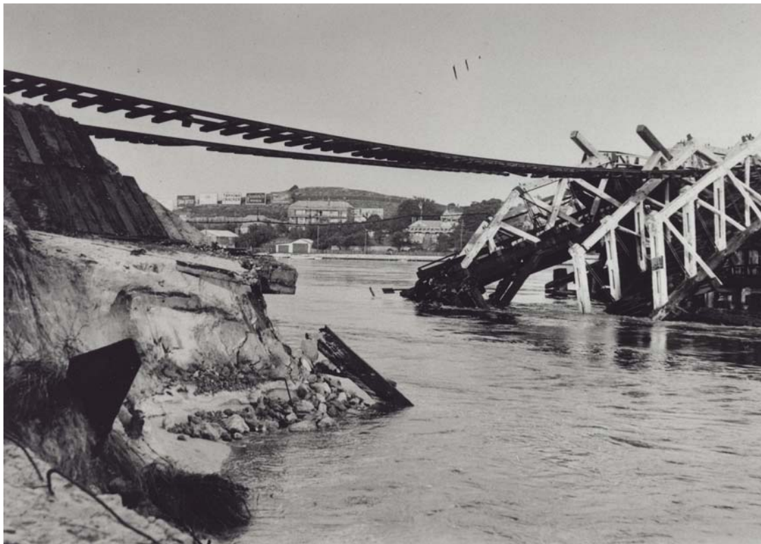
Plate 4.2: Fremantle Railway Bridge destroyed by the July 1926 floods (Courtesy of the Battye Library 54902P)
