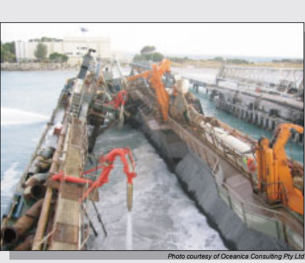
Discharging hopper load of shellsand at Cockburn Cement's wastewater reclaimer
