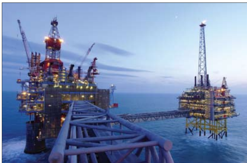
Figure 3. The Sleipner Project in the Norwegian North Sea has injected one million tonnes of carbon dioxide into a sandstone 900 metres below the seabed every year since 1996 (Courtesy of Statoil).
