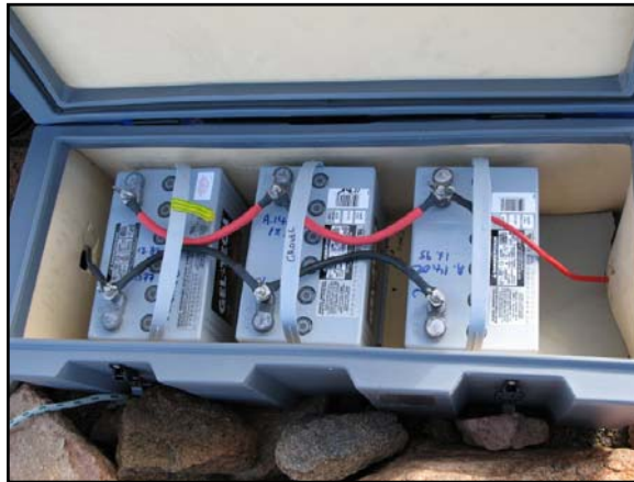
Figure 35: Grove Mountains, inside second battery box.
