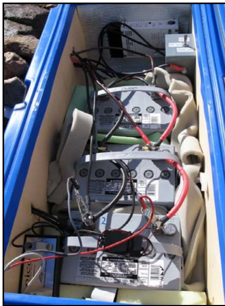
Figure 30: Grove Mountains, inside primary battery box.
