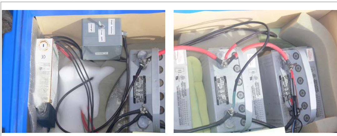
Figure 13 and 14: Wilson Bluff, left and right side of the battery box. Notice the drift snow and corroded terminals.
