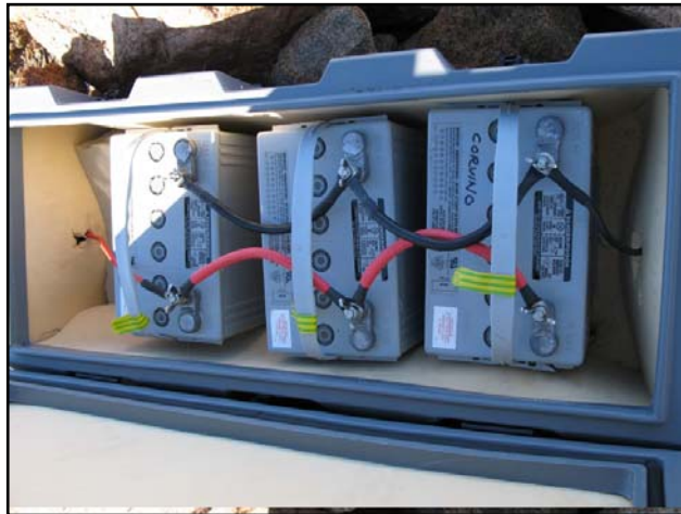
Figure 31: Grove Mountains, inside secondary battery box.
