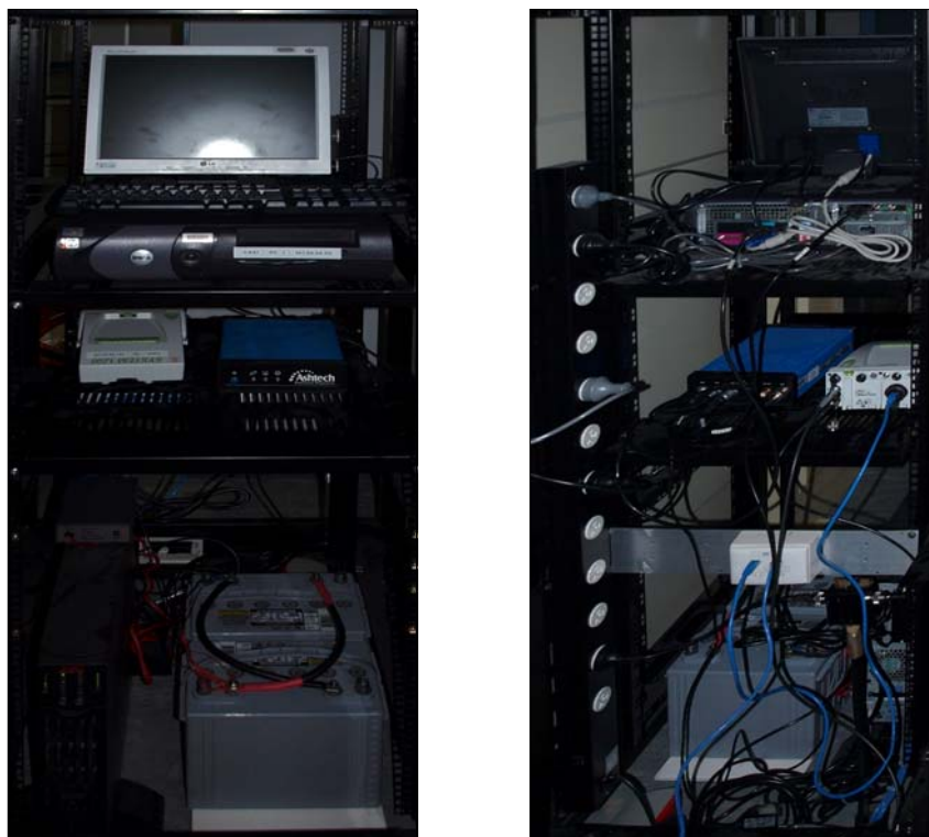
Figure 2: Casey GNSS Equipment Rack from the front (left) and back (right) (December 2008).
