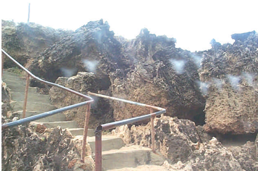
Figure 4.3 Limestone blocks encroaching on to a stair way that provides the public with beach access.
