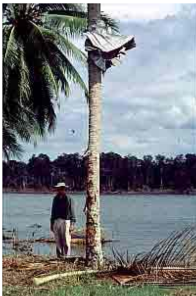
Evidence of the height of the wave, roof sheeting wrapped around a coconut palm.
