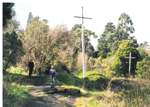
Figure 10: Lumpy topography and tilted telegraph pole following a landslide at Warbuton, Victoria.
