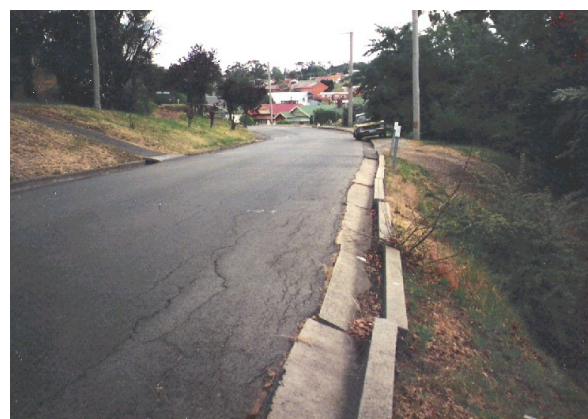
Figure 12: Cracked road and displaced kerb as a result of a landslide in Lawrence Vale, Launceston, Tasmania.
