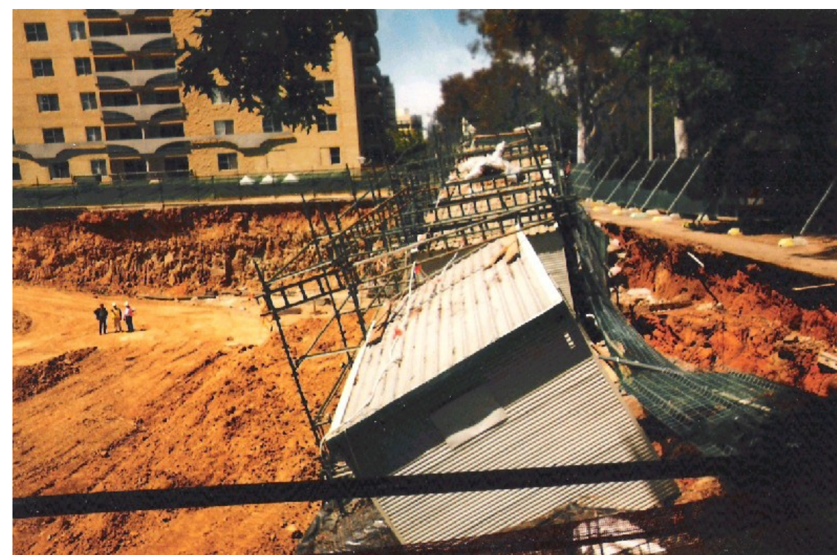
Figure 6: Landslide along the wall of a building site excavation near Northbourne Avenue, Canberra in 2001.
