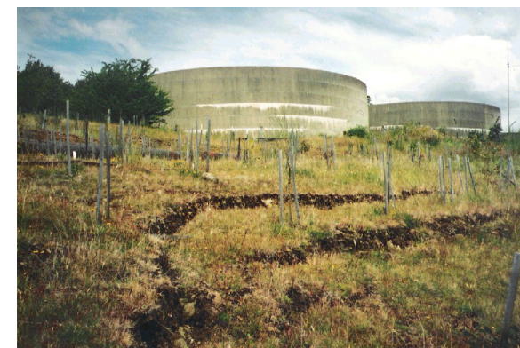
Figure 5: Breaks in the ground at the head of a landslide at St Leonards, Launceston, Tasmania. This landslide was triggered by water leaking from one of the water tanks.
